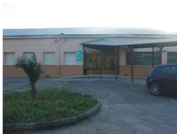
Figure 6.10. Department Pavilion III.
