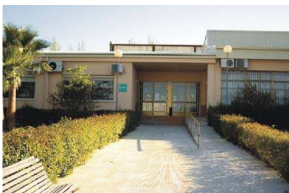
Figure 6.9. Department Pavilion II.
